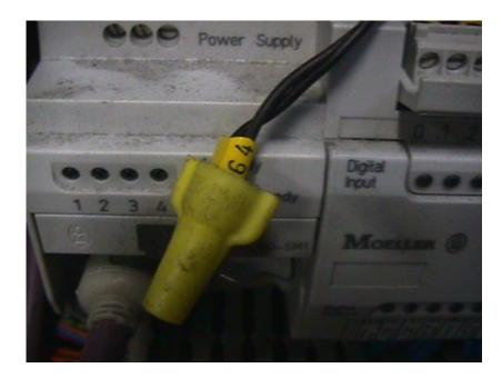
8. Disconnect the Quipp Packman "Downstream interlock" signal wire X1/16 from input I1.0.6.
